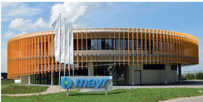
Communications Centre mayr.com – opened in 2018.
